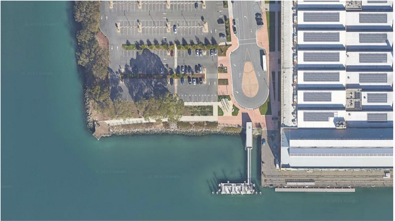
Figure 30: Aerial Image of Richmond Terminal Credit: Arup
